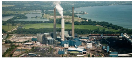
Monroe power plant | Port of Monroe
