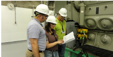
NRC inspectors conduct seismic walkdowns at the Kewaunee nuclear plant. | NRC
