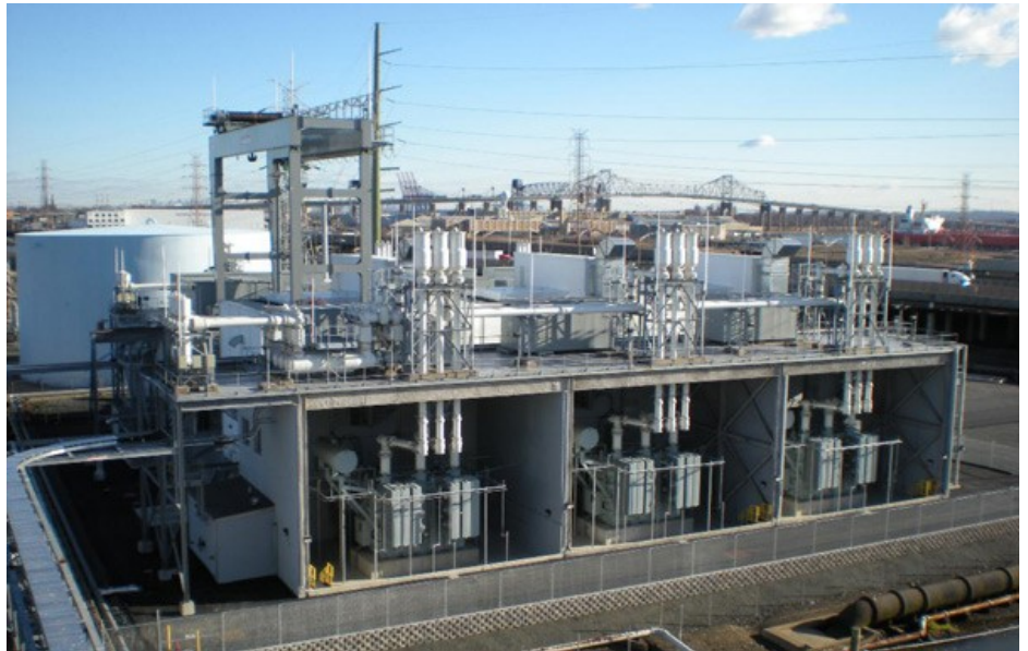
Linden VFT facility | Joseph Jingoli & Son
